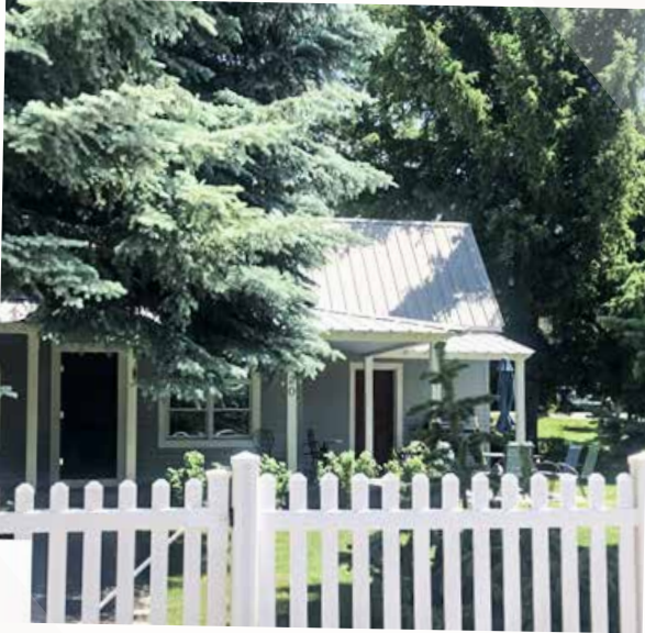
2nd Avenue House in Hailey, Idaho
